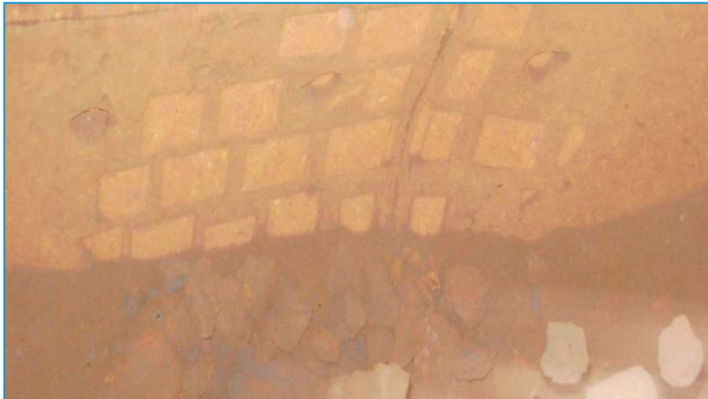
TEGA MOSAIC LINERS INSTALLED IN CHUTE HANDLING IRON ORE LUMPS
