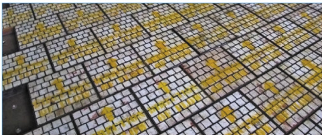
Screen underflow chute lined with D-Mac Ceralock
