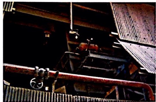
Installation on a Discharge Chute
